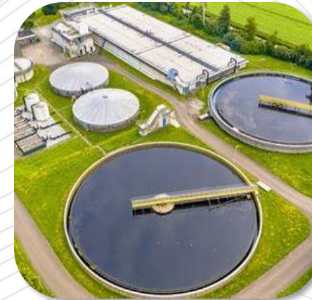
Sewage treatment system
